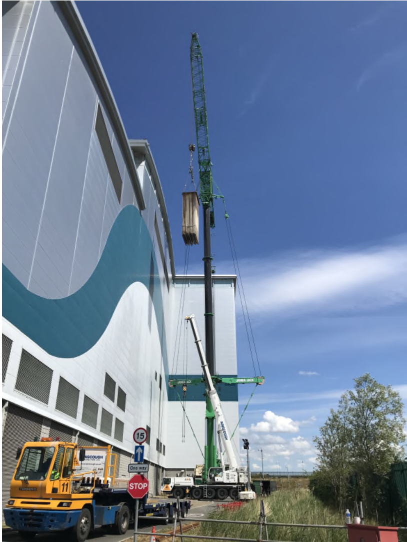
Figure 1 Crane on eastern side of Riverside 1, looking north
